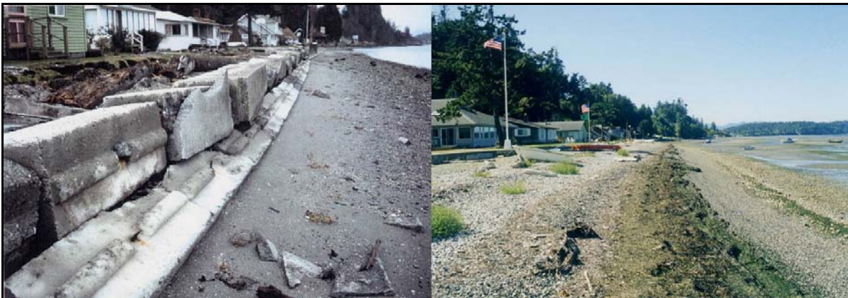
Figure 17: Before and After Shoreline Restoration, Washington
